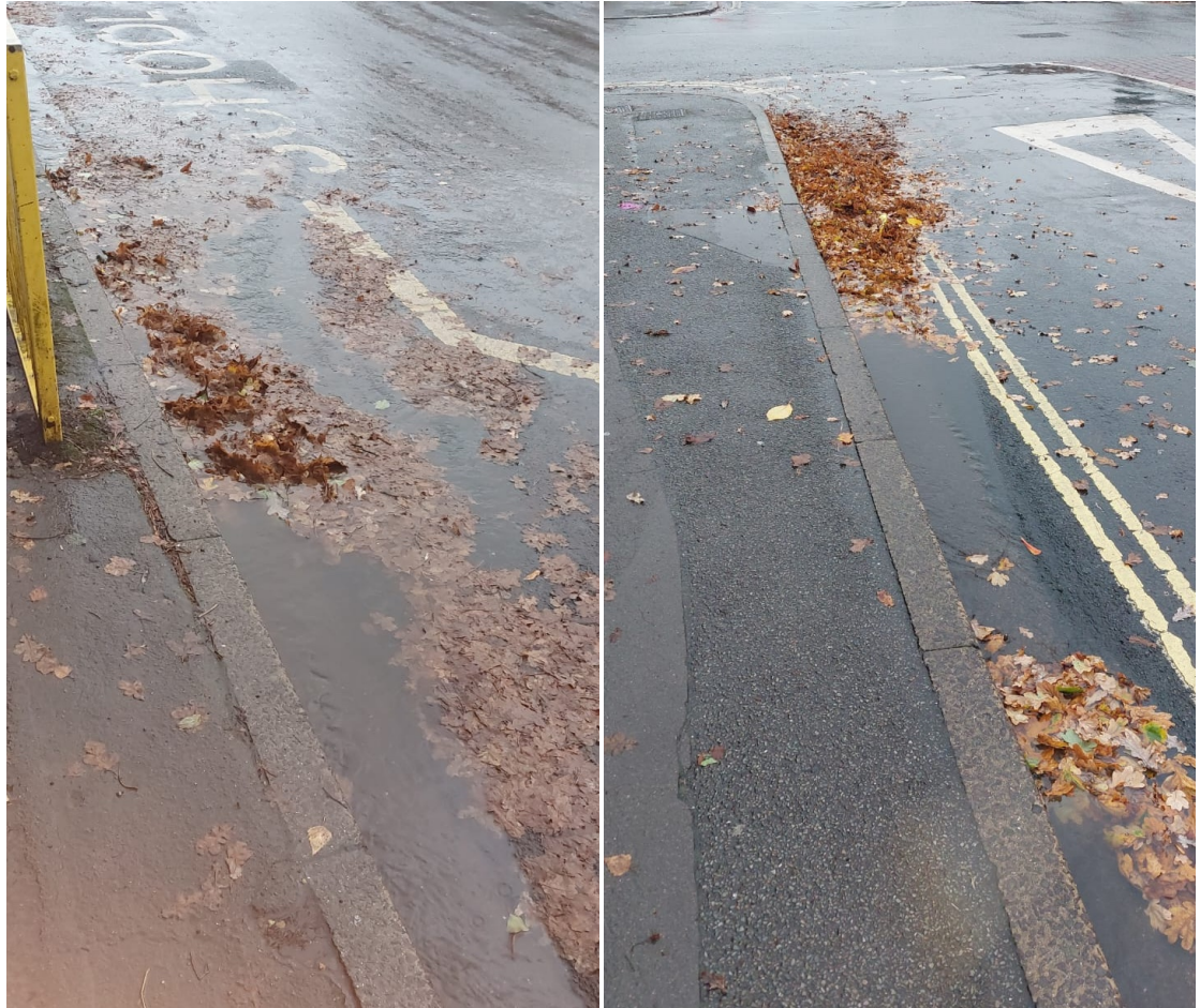
Figure 6. Examples of flooding due to debris on Mayfield Road.
